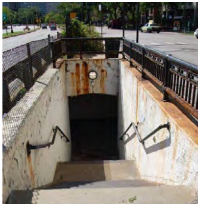
Exhibit 2-4: Existing Pedestrian Underpass
