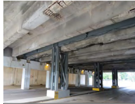
Exhibit 2-3: Temporary Bridge Supports
